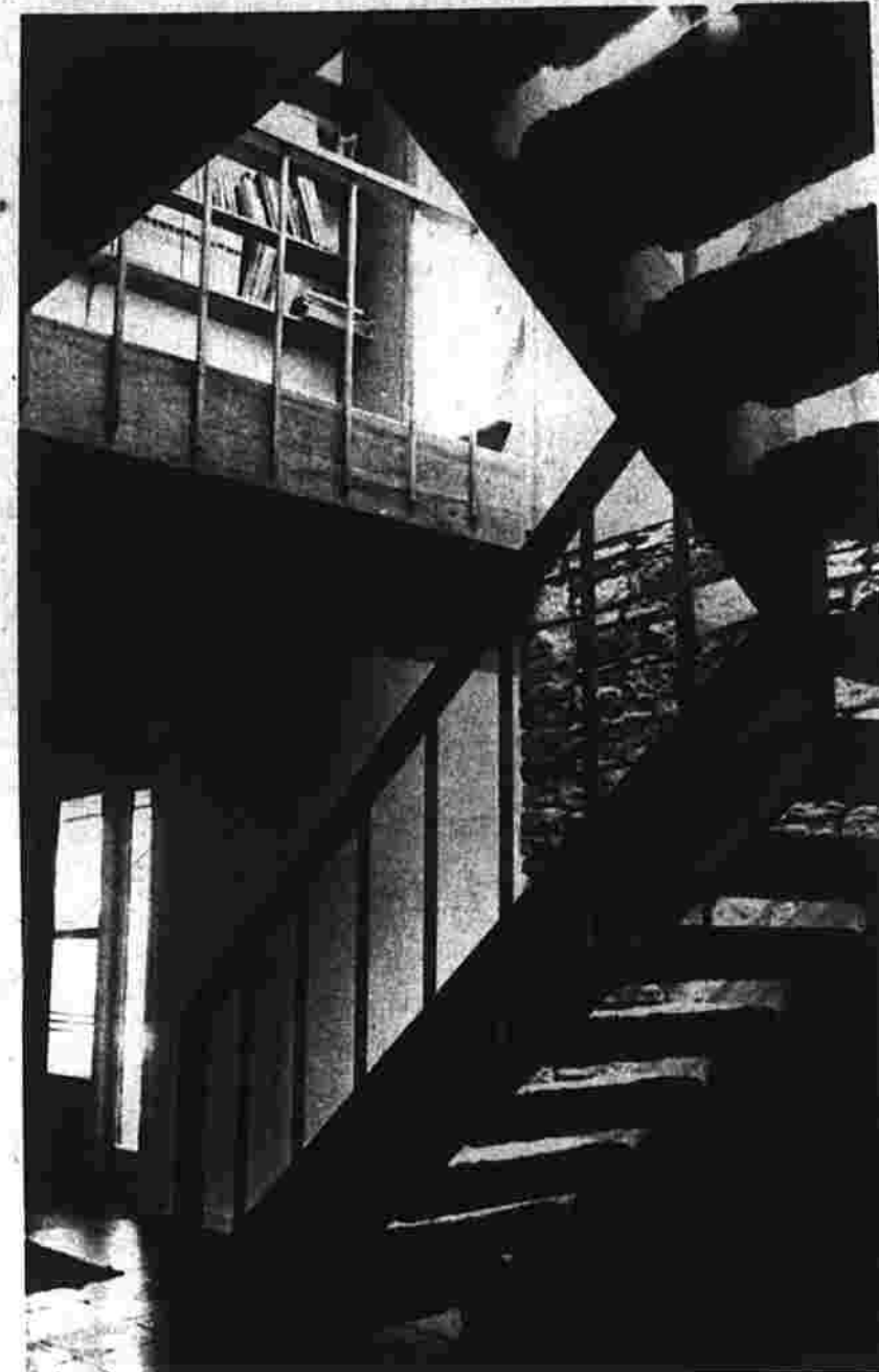
Floating stairway, brightly illuminated by skylight, dominates foyer.
